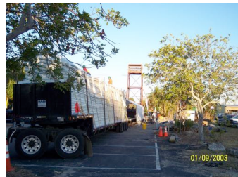
Liner positioned on jobsite at the beginning of the Wetout facility
