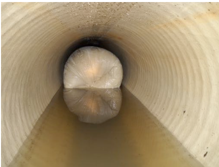
(Photo: 24" being installed thru 30" CIPP)
